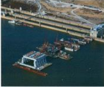
Pictured above is the Olmsted Locks and Dam.
