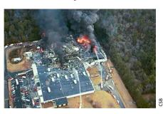
On Jan. 29, 2003, an explosion and fire destroyed the West Pharmaceutical Services plant in Kinston, NC, causing six deaths, dozens of injuries and hundreds of job losses. The CSB report found that the fuel for the explosion was a fine plastic powder, which accumulated above a suspended ceiling over a manufacturing area at the plant and ignited.
